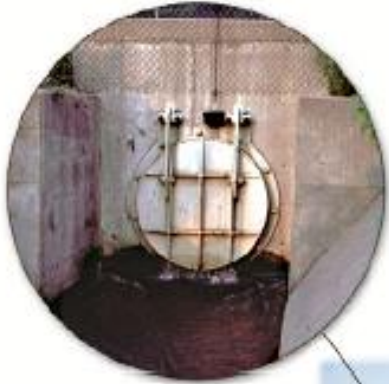
Combined Sewer Overflow
